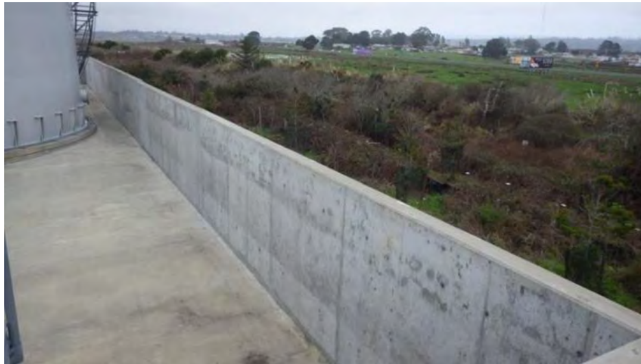
Figure 7. Existing HBGS containment wall.
