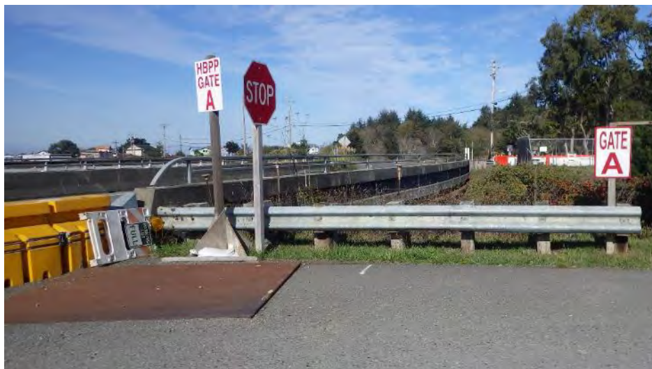
Figure 8. Existing W-beam guardrail between Intake Canal and Alpha Road.
