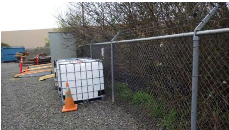
Figure 6. Existing HBGS fencing.
