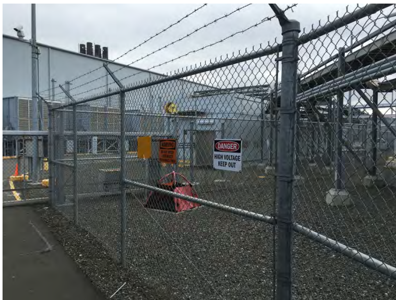
Figure 5. Example of existing switchyard fencing.
