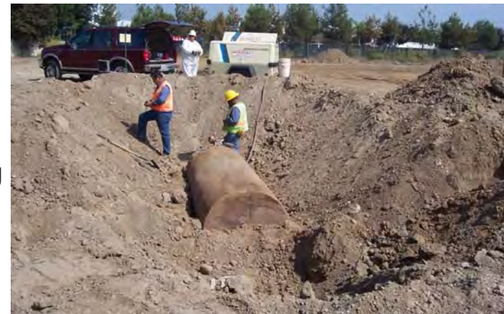
Unexpected clarifier and underground storage tank requiring excavation and removal.
