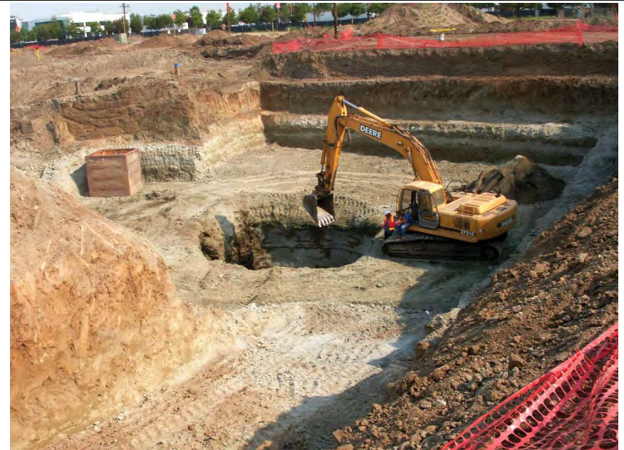
Large excavation to abandon deeply buried oil well.
