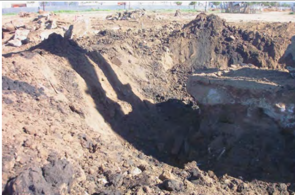
Removal of a Concrete Footer Used for Oil Rig Tie-Down
