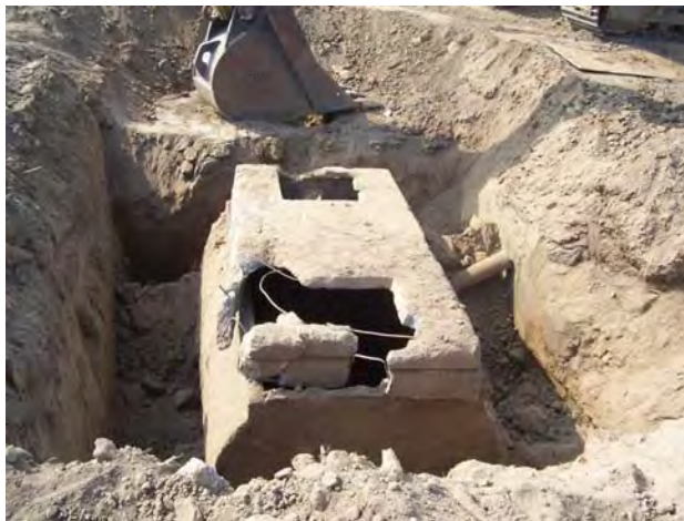
Removal of a Concrete Footer Used for Oil Rig Tie-Down
