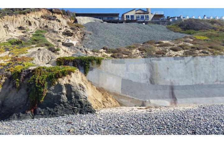
Photograph taken in January 2016 and provided to staff by the applicants. Applicants state that 29 ft. of the 50 ft. long seawall on the subject site is fronted by landslide deposits.
