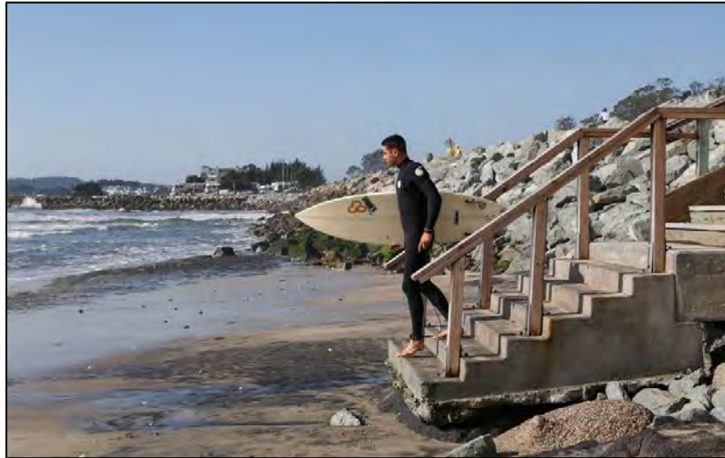
A surfer uses the repaired beach access stairs at Surfers Beach in Half Moon Bay.
