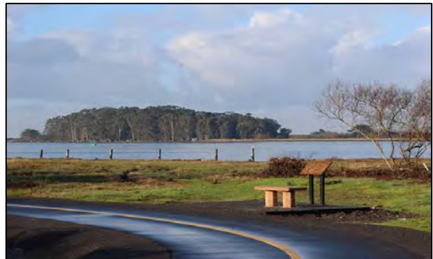
New Section of the Coastal Trail along Humboldt Bay in Arcata and Eureka are part of a major Highway 101 improvement project.
