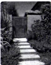
Grass Paver Block Walkway Photo Credit: City of Los Angeles
