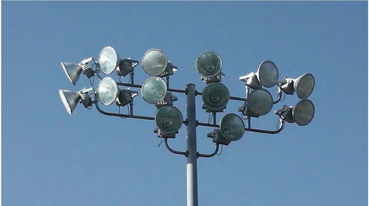
ROB FIELD 4 – MUSCO METAL HALIDE ‘LIGHT STRUCTURE GREEN’
