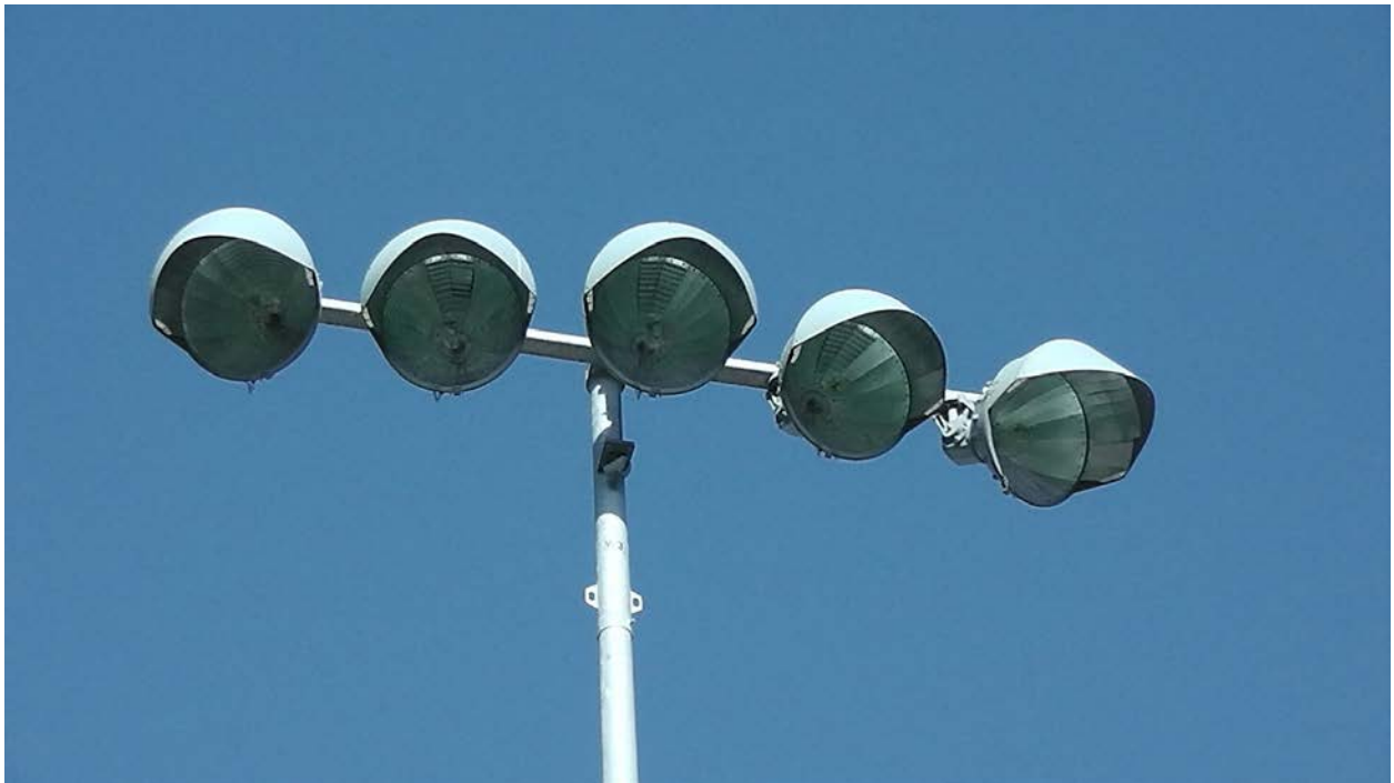
ROB FIELD 4 – MUSCO METAL HALIDE ‘LIGHT STRUCTURE GREEN’
