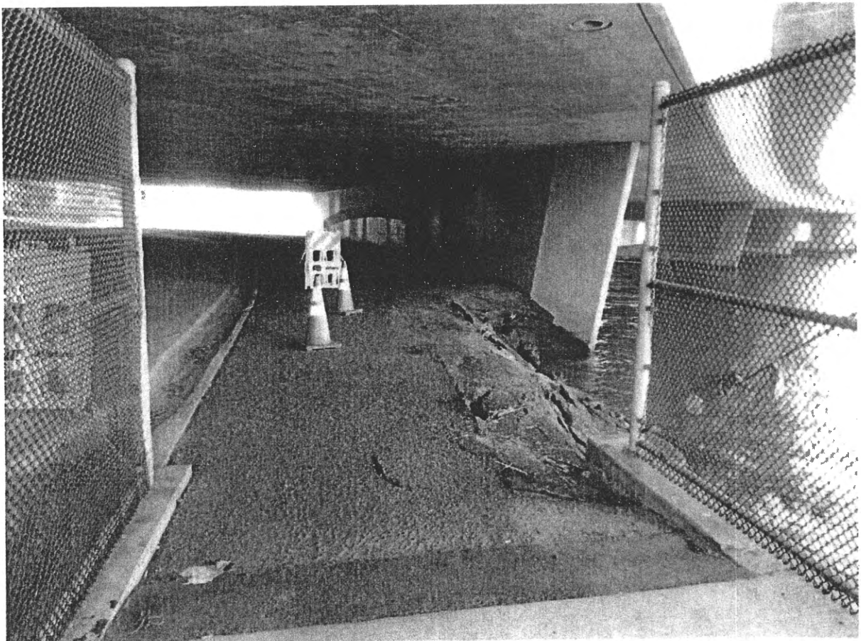
Figure 3. Failed Section of the Bike/Pedestrian Path
