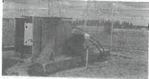
Fig. 2. Distribution Personnel Installing Padmounted Substation
