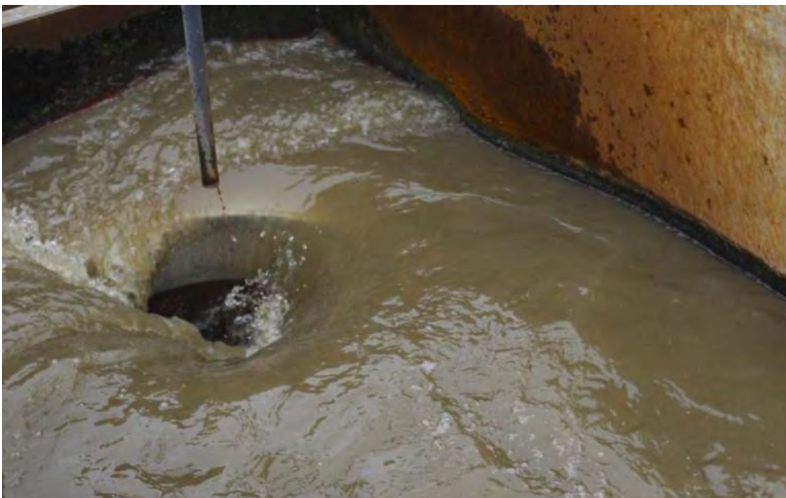
A grit-removal system will help prevent buildup in the digester at the Oceano wastewater treatment plant.
