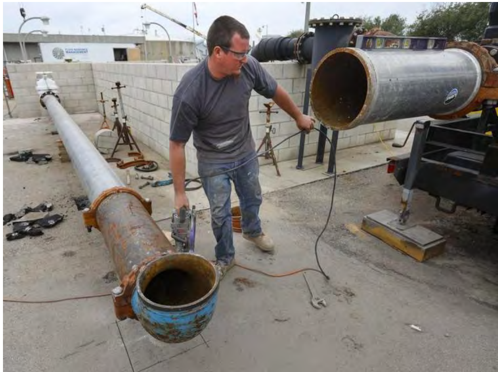
Jack Early prepares pads for concrete pipe stands. The 12-inch emergency bypass pipe is being moved to accommodate upgraded equipment. The South San Luis Obispo County Sanitation District has had an expensive year for capital projects as its board tries to update its 50-year-old wastewater treatment plant in Oceano.
