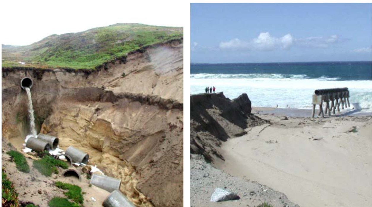
Figure 5: Erosion exposing storm drain outfalls on Former Fort Ord
