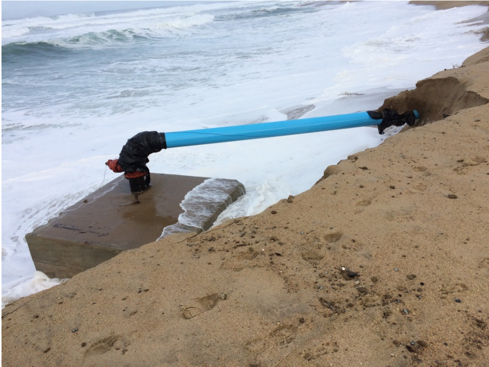
February 20, 2016 – Erosion undercutting regional sewage outfall (cement block) and Cal-Am test well discharge (blue pipe)
