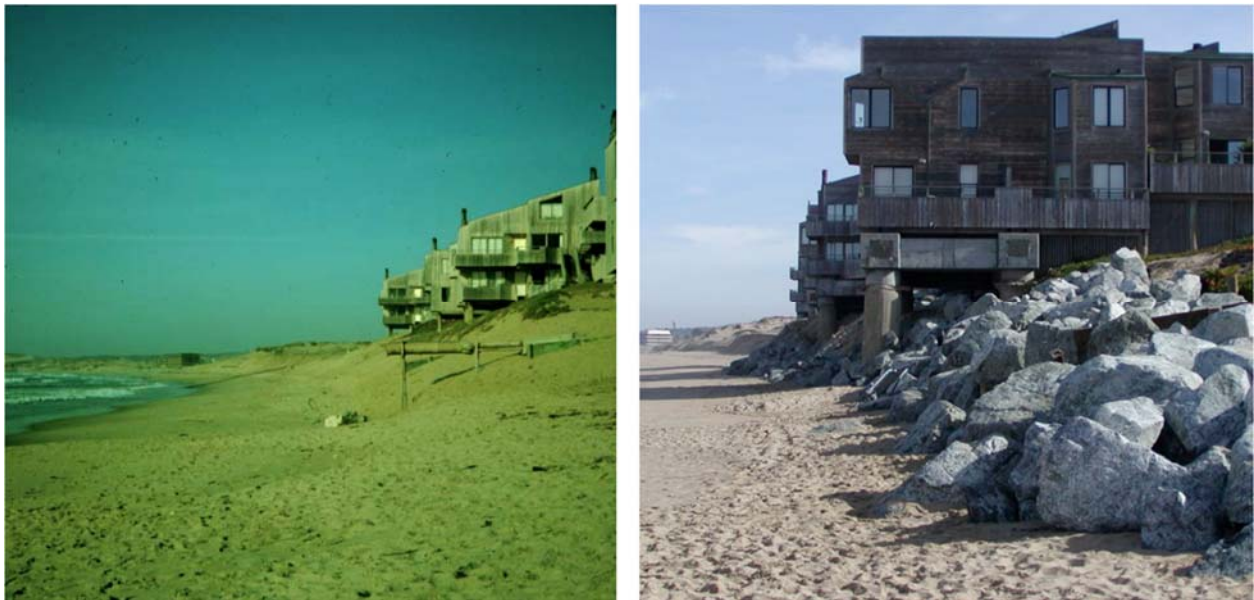
Figure 2: Erosion in front of Ocean Harbor House Condominiums
