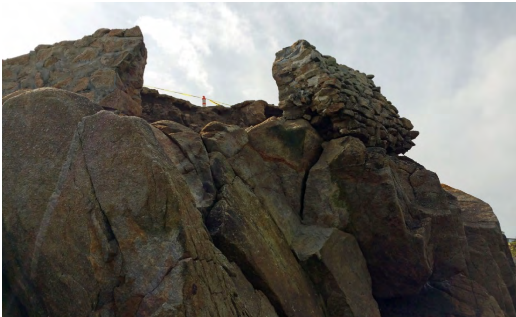
Photograph 3: Showing Failed Area of Existing Coastal Protection and Precarious Wall Segment at Top of Bluff
