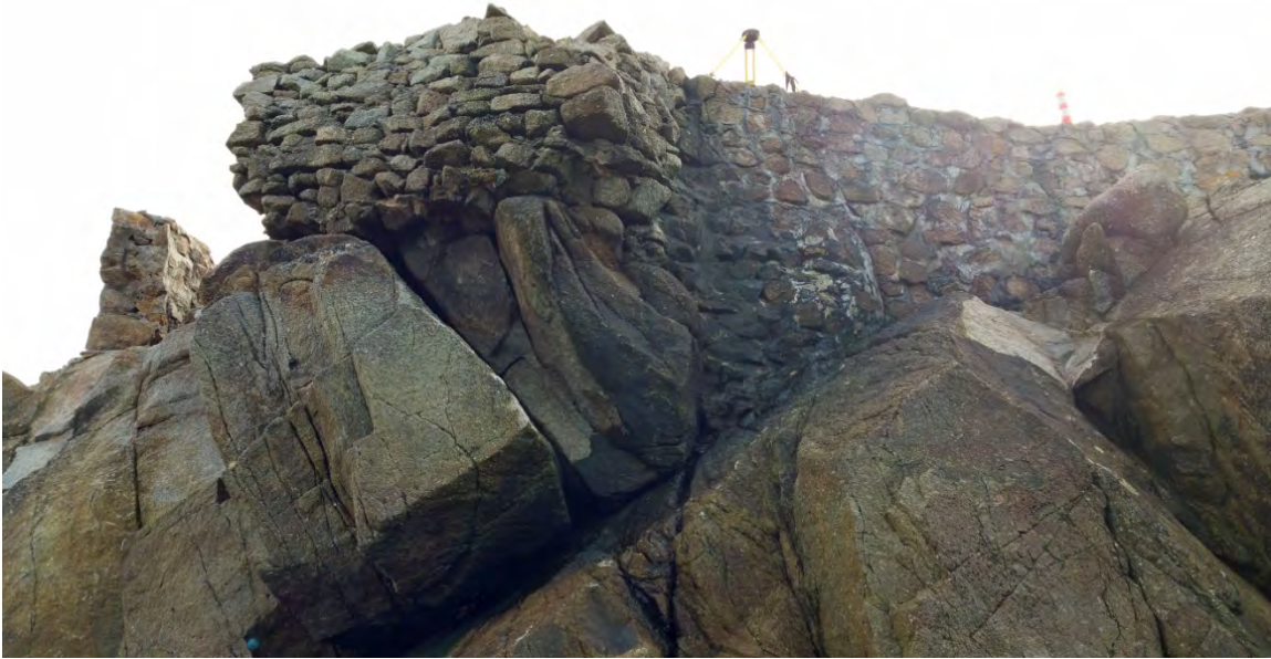
Photograph 6: Showing Precarious Portion of Wall in Relation to Stable Part of Wall at Downcoast Area of Overlook Bedrock in Left Half of Photo is Unstable
