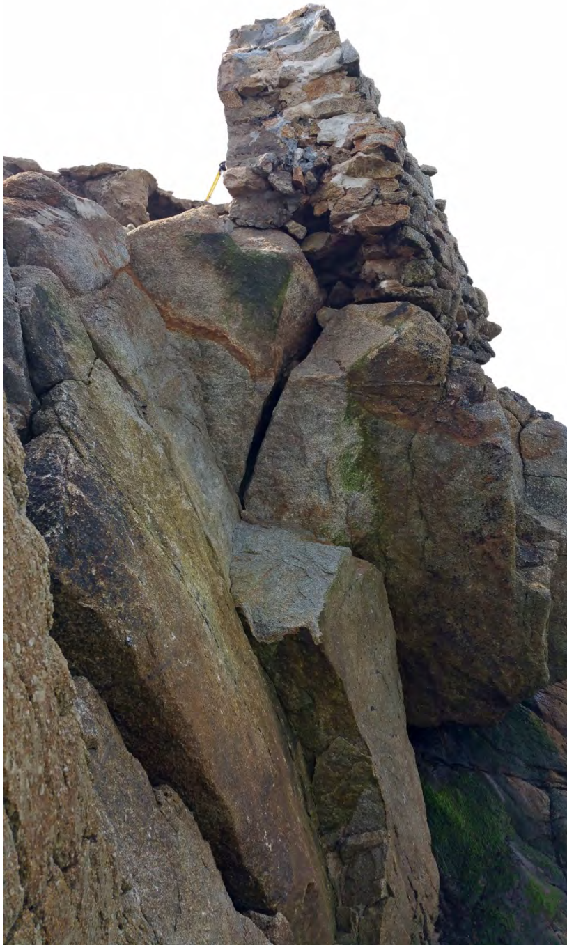
Photograph 4: Showing Cracked Bedrock Below Wall And Recent Bedrock Failure Area That Damaged Wall
