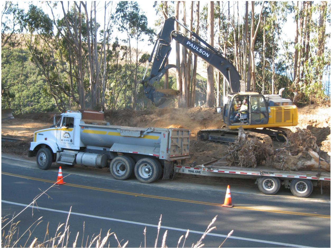
EXHIBIT 3. 20181015-1100. Caltrans-contractor's bulldozer grades the northerly edge of the north staging area (southerly subarea 1), without erosion control/water quality BMPs. Photo orientation: Looking southwesterly across canal-off Highway 1 to the remaining trees on the Albion Cove coastal bluff (on the private Seto property).
