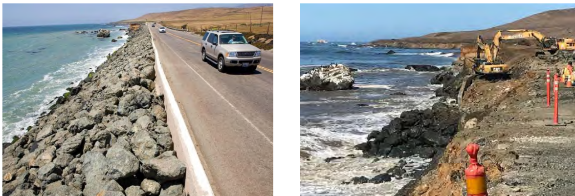
Highway One at Piedras Blancas realignment and revetment removal – before and after.
