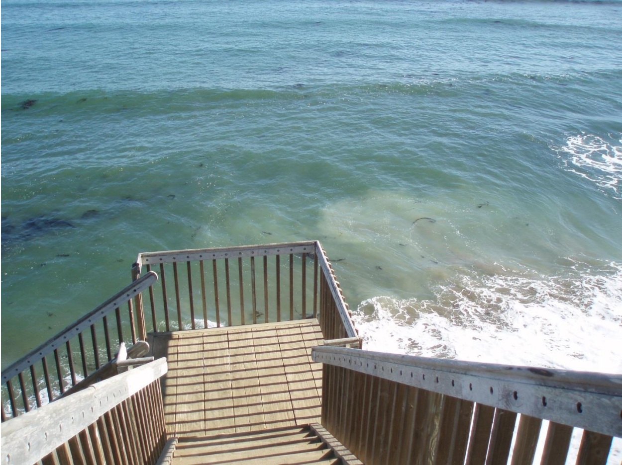
Beach Access Stairway:
