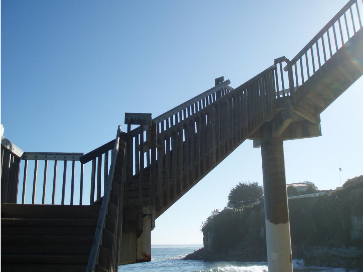
Beach Access Stairway:
