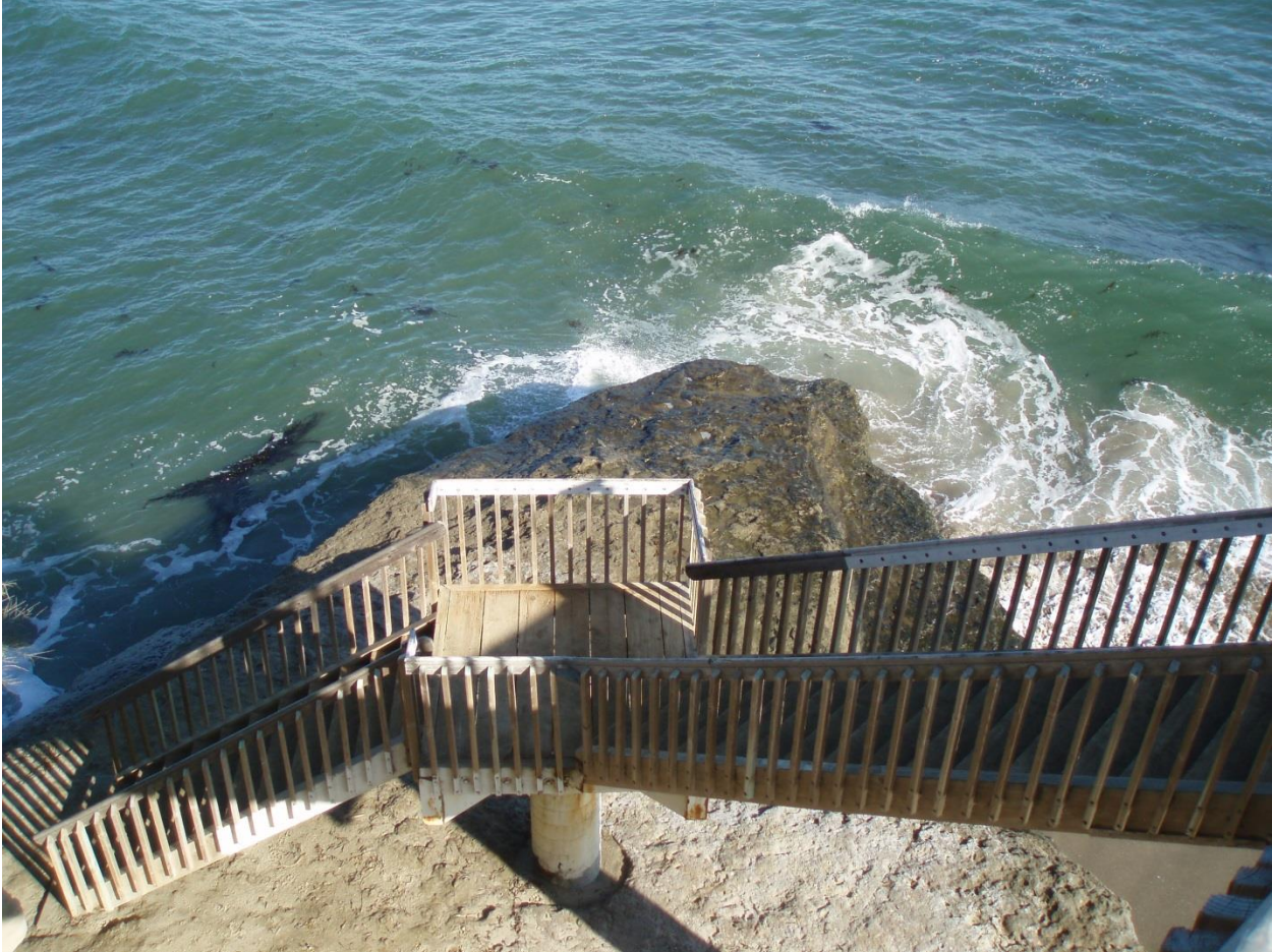
Beach Access Stairway:
