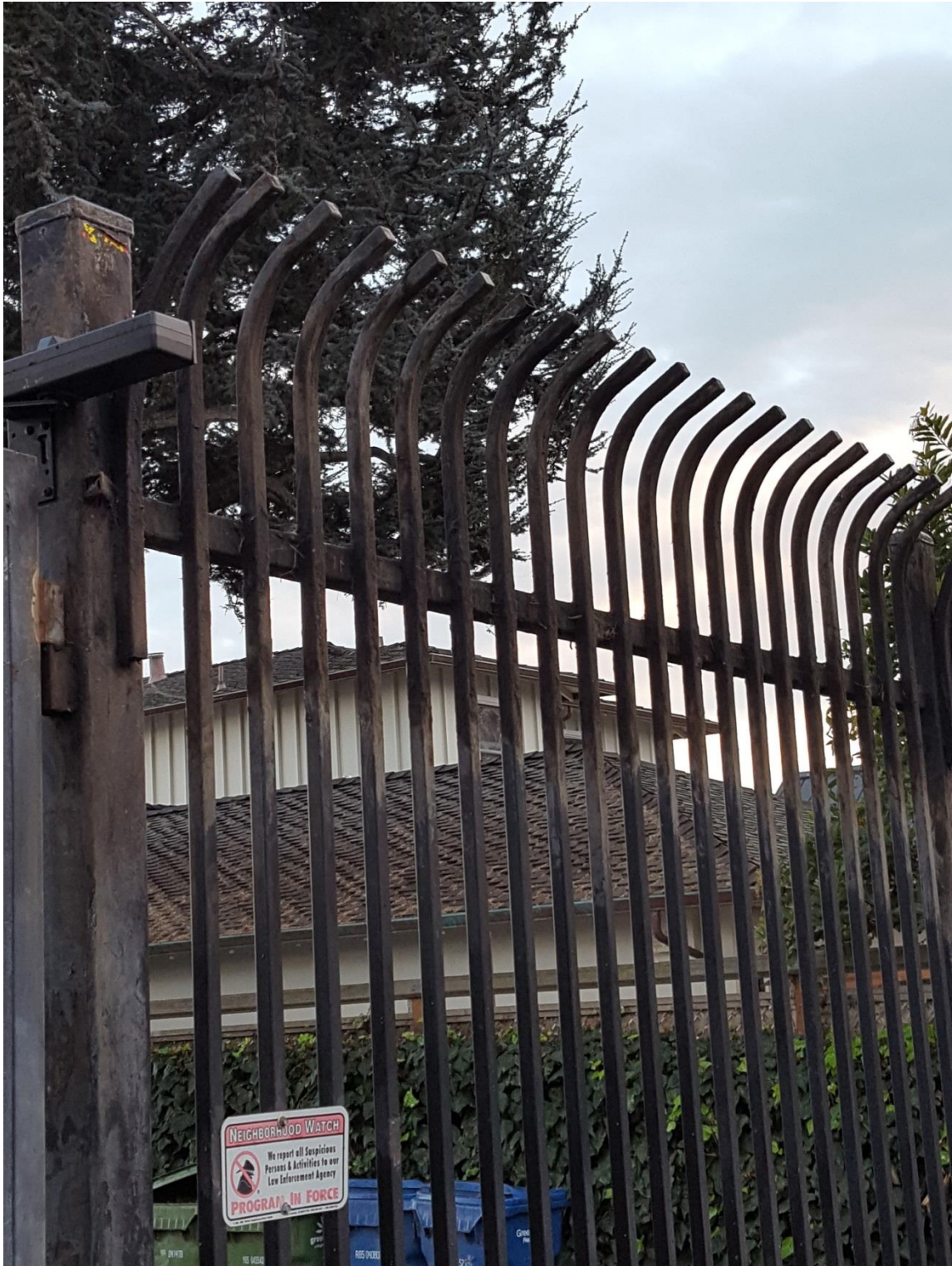
Top of Nine-Foot Tall Wrought-Iron Fence:
