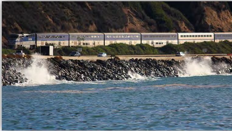
Figure 7. Photo of infrastructure at risk near Rincon Beach, Ventura, CA, during the King Tide in December 2012. (Photo courtesy of David Powdrell, California King Tides Initiative)
