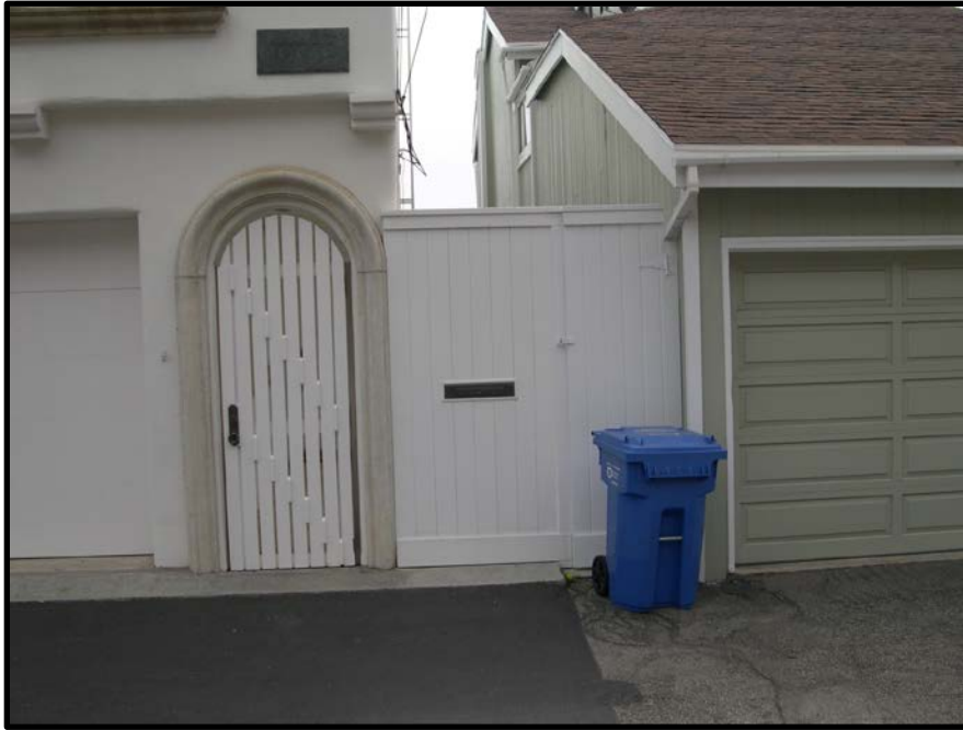
(Exhibit 8: Public access violations can involve unpermitted development that physically obstructs access, such as this locked gate, blocking a public access easement.)
