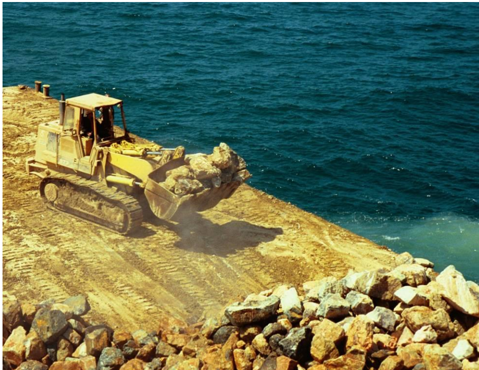
Figure 6-2. Rock placement method: front-end loader/flat supply-barge “push off” method.
