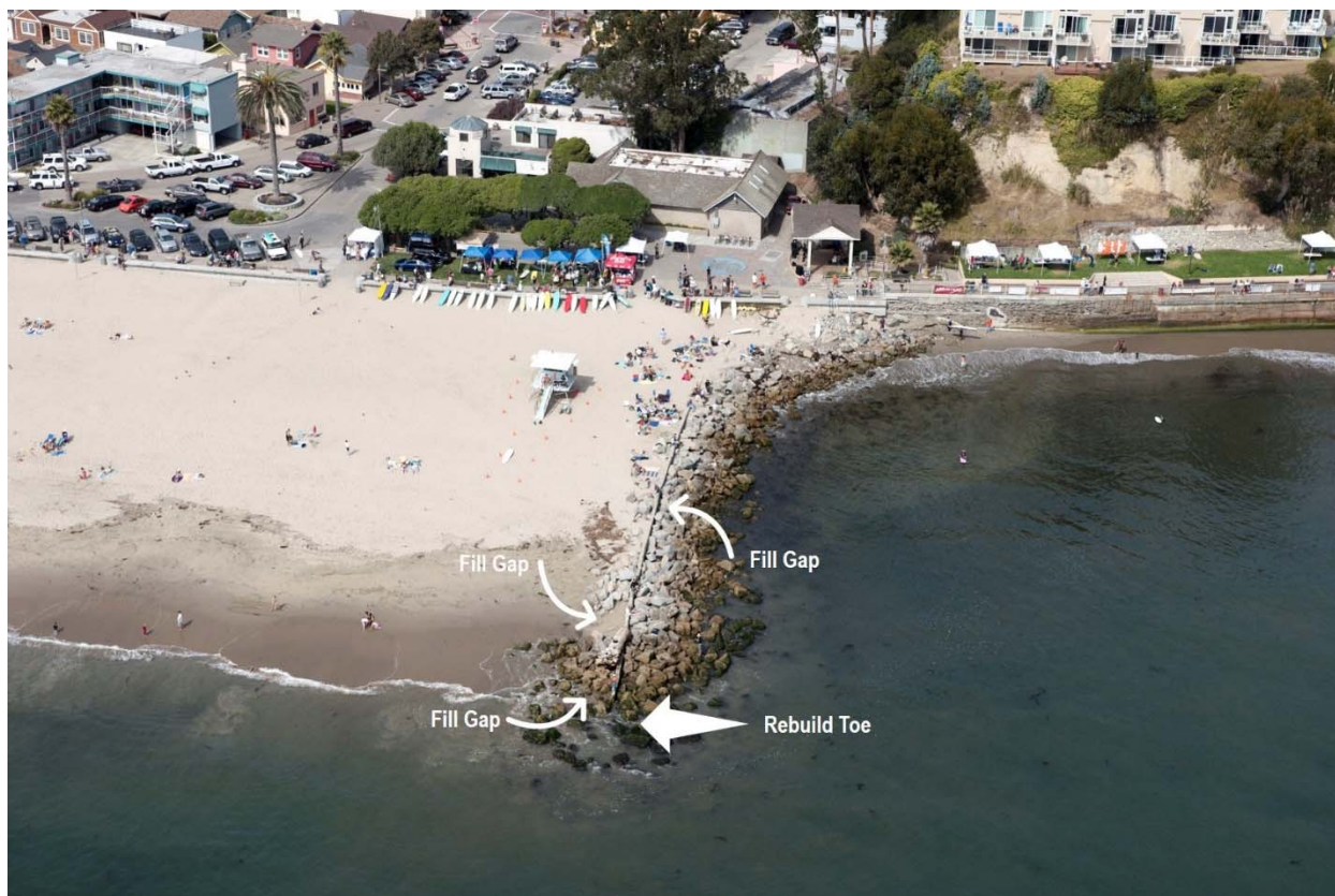
Figure 3: Proposed Repairs to Jetty
