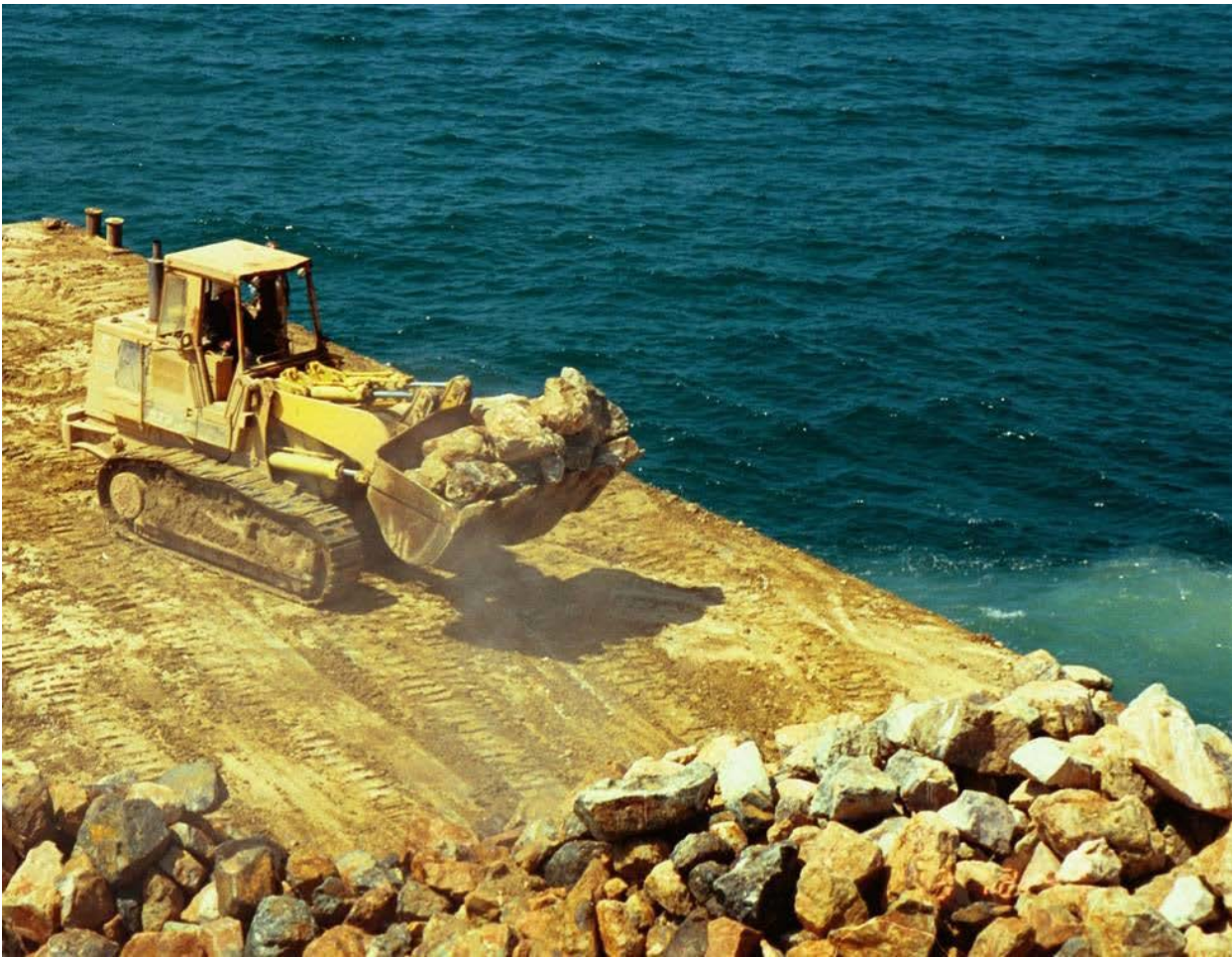
Front-end Loader Pushing off Rock Boulders for Reef
