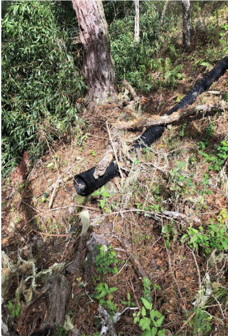
End of motor court discharge pipe at bottom of ravine on Applicant's property. New energy dissipators will be located at outlets of each existing pipe on Applicant's property (County photo)
