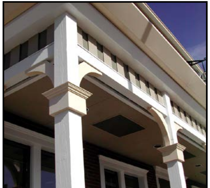
Appropriately sized and functional column
