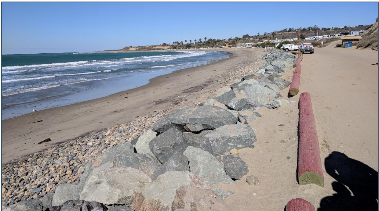
FIGURE 3.8: EMERGENCY REVETMENT APPROXIMATELY ONE YEAR LATER, MARCH 2018
