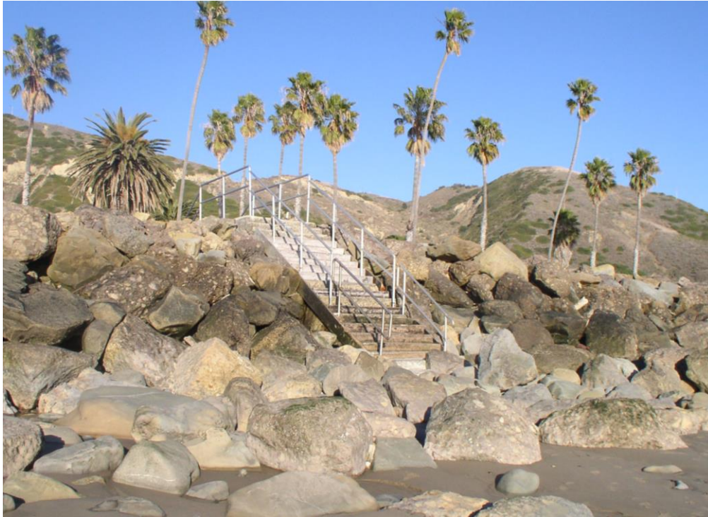
FIGURE 8.2: EXAMPLE REVETMENT STAIRS – AT HOBSON COUNTY PARK IN VENTURA
