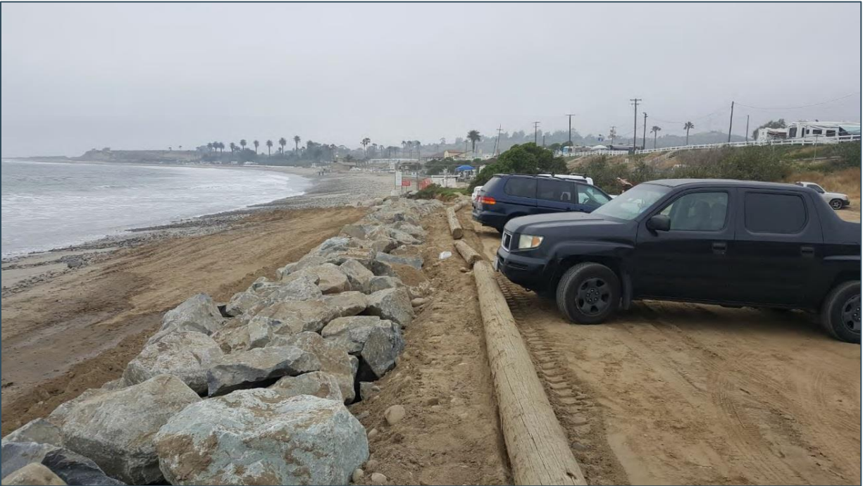
FIGURE 3.7: EMERGENCY ROCK REVETMENT IMMEDIATELY FOLLOWING CONSTRUCTION, MAY 2017 (CCC)
