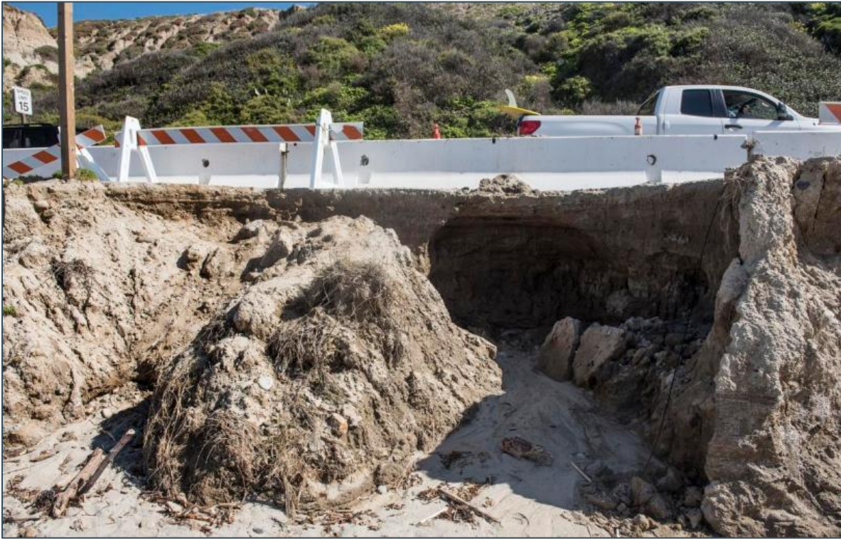
FIGURE 3.4: UNDERMINING OF ROAD/PARKING AREA FROM 2017 STORM DAMAGE (OC REGISTER, 2017)
