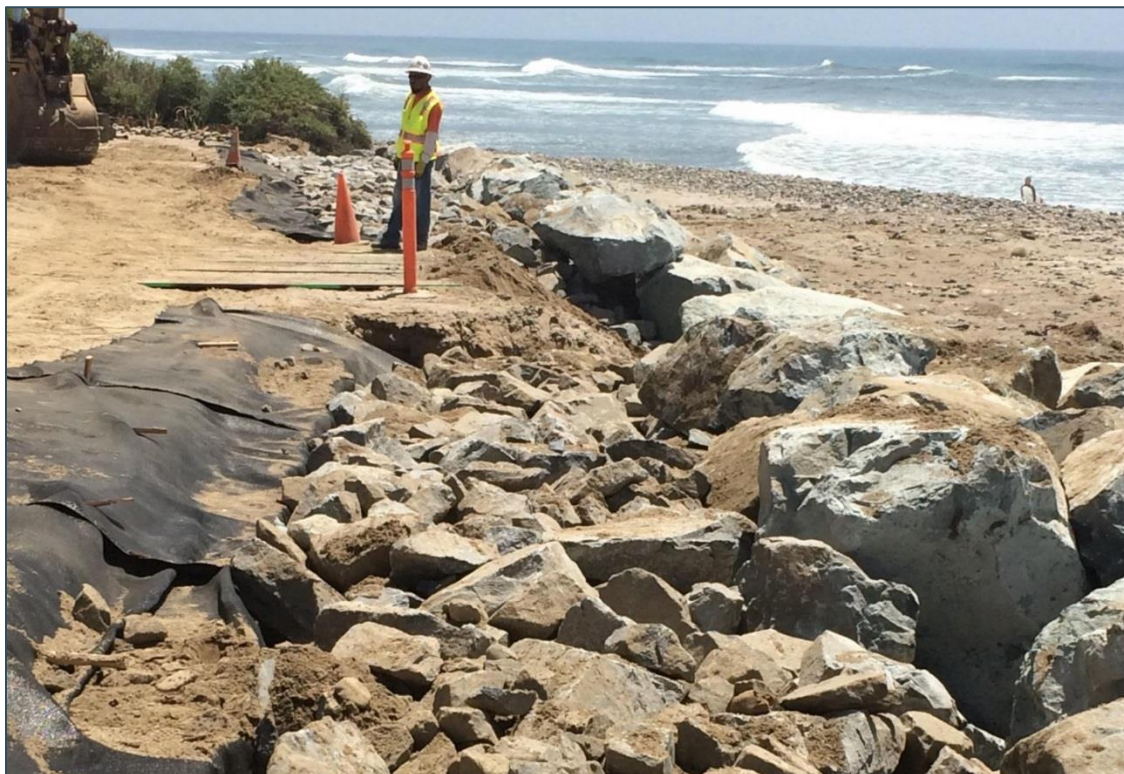
FIGURE 3.6: CONSTRUCTION OF EMERGENCY ROCK REVETMENT, APRIL 2017 (SURFRIDER, 2017)
