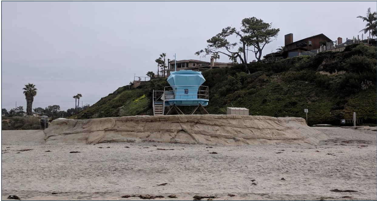
FIGURE 8.4: SCULPTED SEAWALL AT CARDIFF STATE BEACH (EXAMPLE OF NARROW FOOTPRINT ARMORING)
