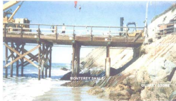
Photograph 3. Gaviota Pier March 2000
