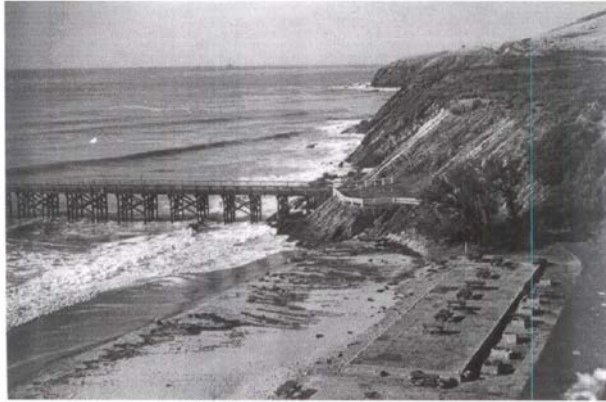
Photograph 2. Gaviota Pier Abutment circa 1974 taken from RR trestle.
