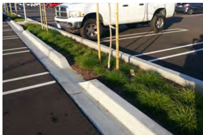
A bioswale in a parking lot can help to reduce stormwater runoff.
