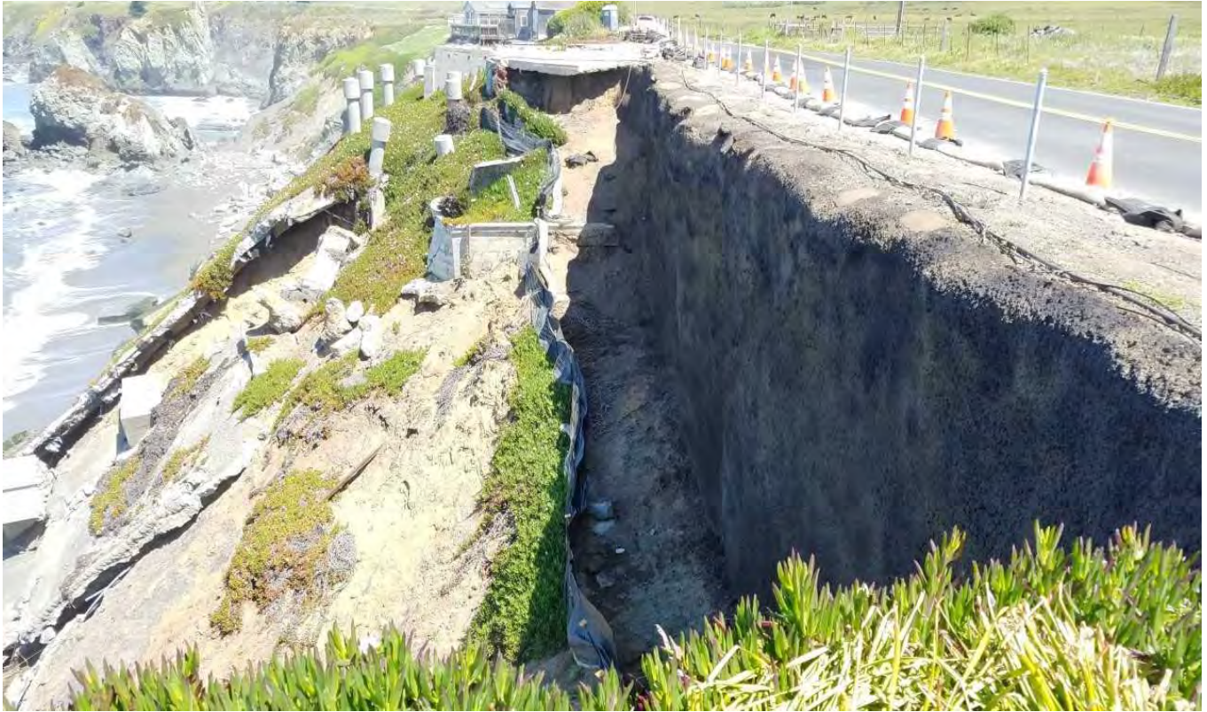
Caltrans 2017 Shotcrete Wall and Sluffing Debris along Highway 1, Bluff Face and Shoreline
