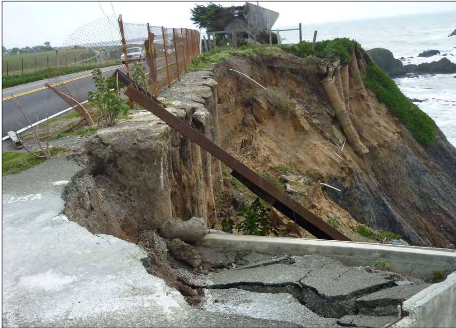
Photo 1. Exposed piles and pavement failure, facing south (March 2010)
