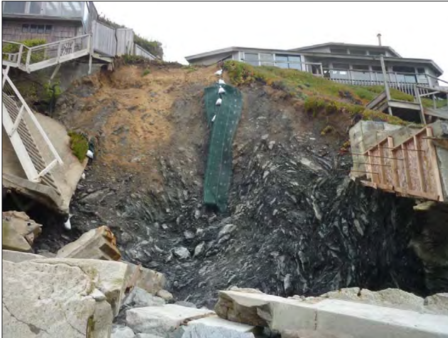
Photo 5. Evidence of recent slope erosion and undercutting of stair structures, facing east (March 2010)
