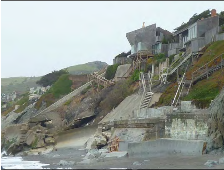
Photo 8. Gleason beach seawalls and slope protection, facing northeast (March 2010)
