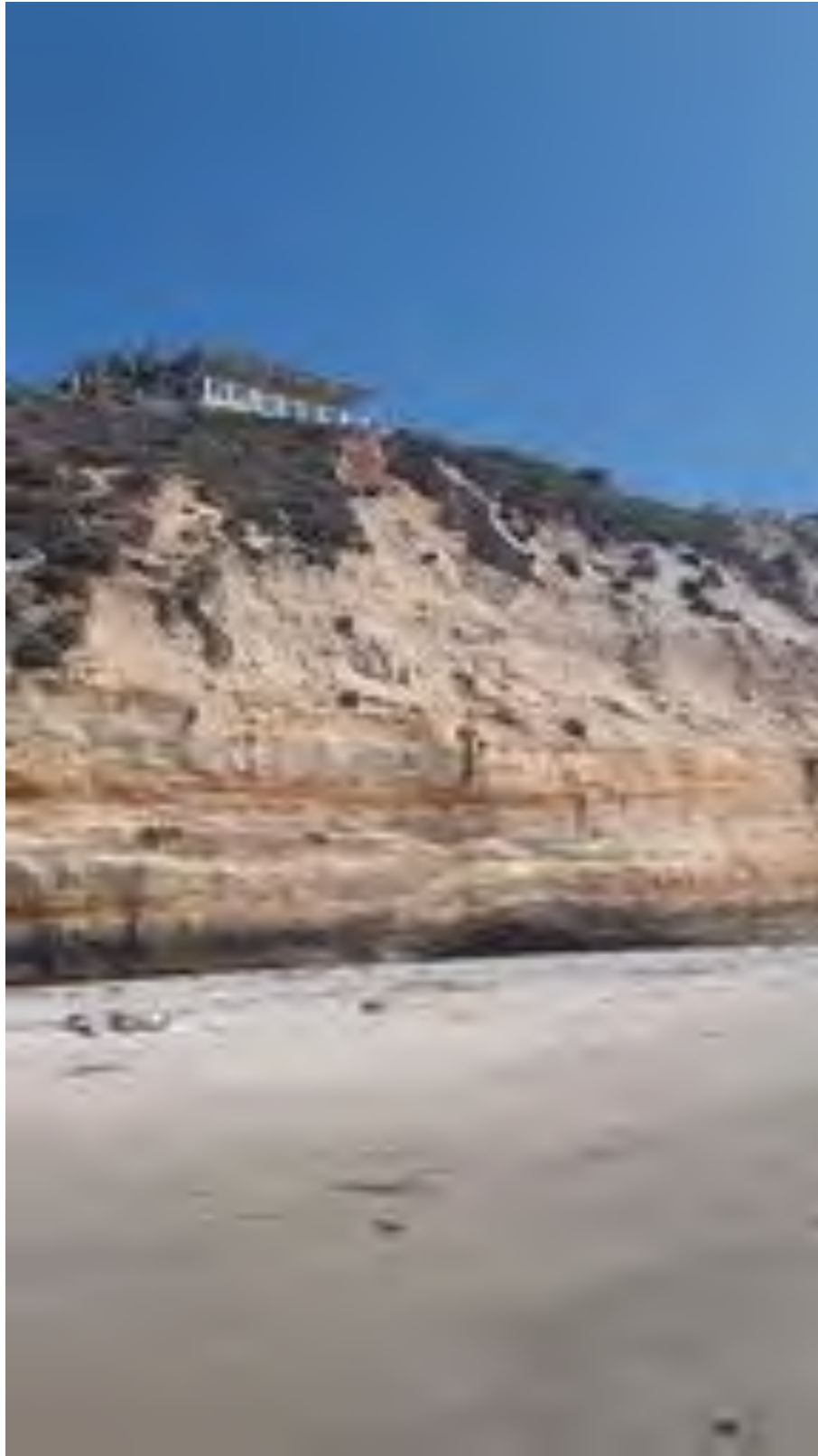
Figure 5: Upper bluff failure example A.
