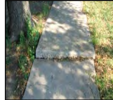
Surface roots have raised the sidewalk.
