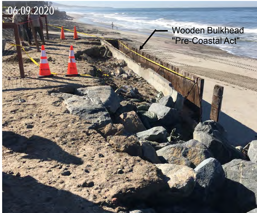
Additional site erosion following removal of boardwalk, basketball court and restroom
