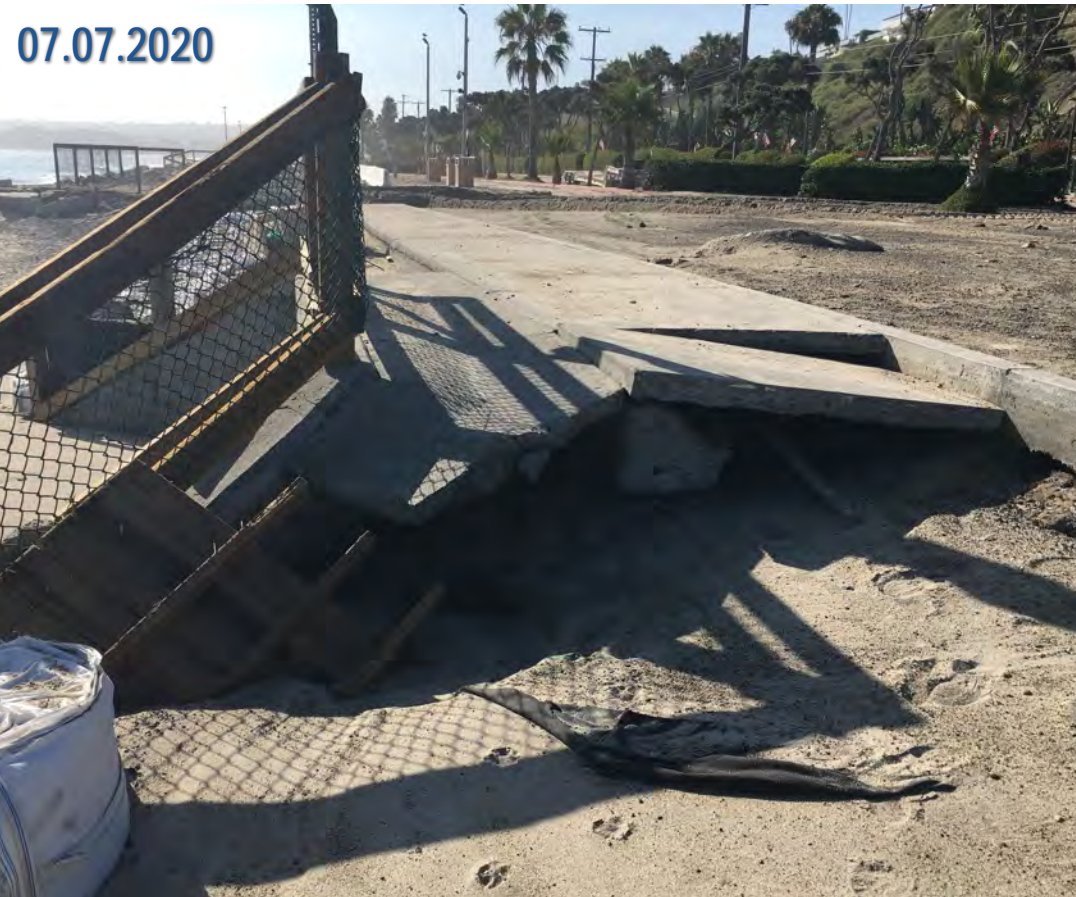
Additional site damage from wave overtopping following sandbag installation
