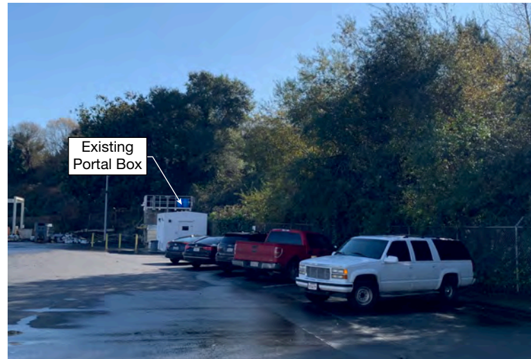
Photo 8 - SC WWTF portal box which will provide connection between the proposed reverse osmosis concentrate pipeline (see Figure 2) and the existing 72-inch-diameter tunnel to ocean outfall, as viewed from within the SC WWTF perimeter fencing, looking southeast.
