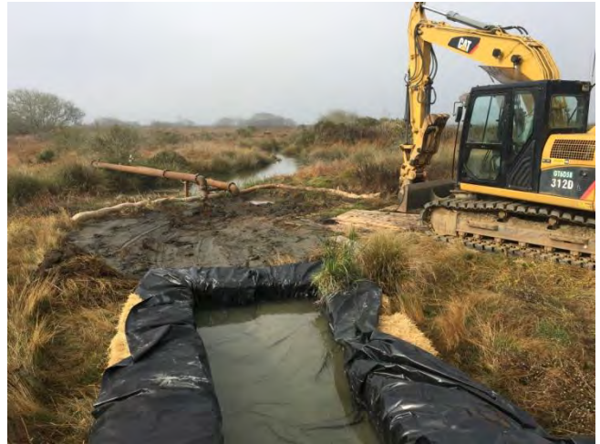
Photo 2. Dewatering settling and infiltration basin.
