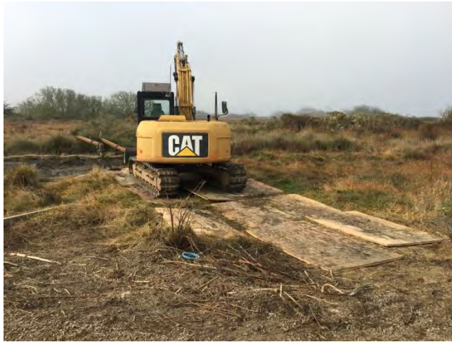
Photo 1. Surface stabilization technique
