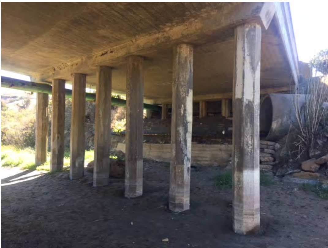
View of existing northbound bridge piles and RSP looking up Toro Creek (top) and south (bottom).
