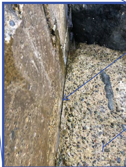
Little to separation between wall panel and concrete base
