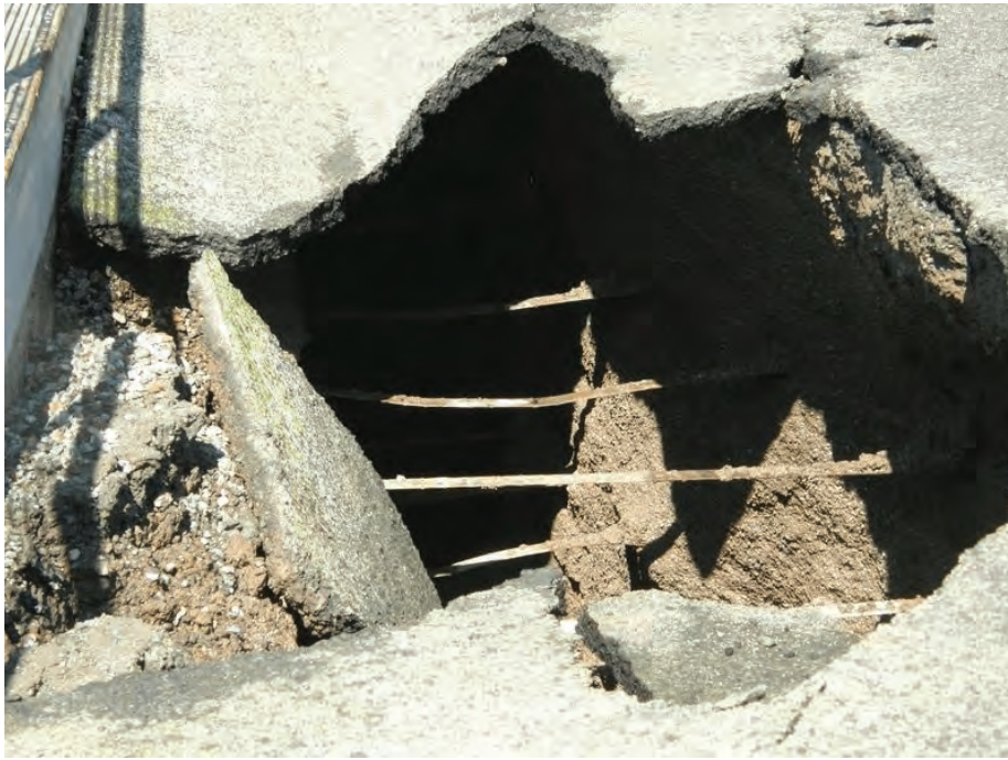
Figure 1. RE wall restraining straps in excellent condition after the 2008 loss of RE wall backfill.
