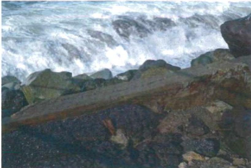
Seawall is nonexistent. At the end of the road damaged storm drain retaining wall abuts RE wall to south.
