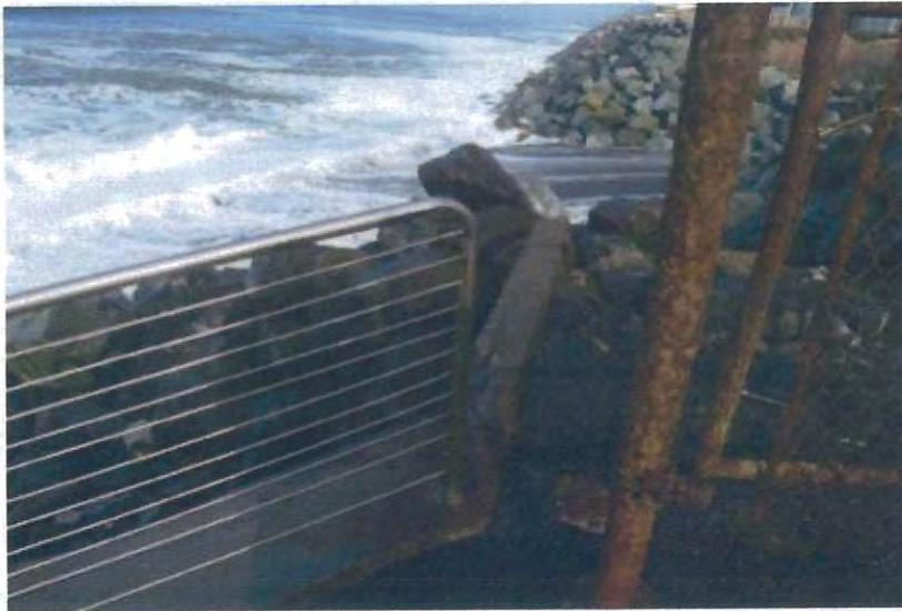
NO seawall exists at the end of Beach Boulevard. Concrete extending north from the RE wall is the facing for the storm drain outlet.
