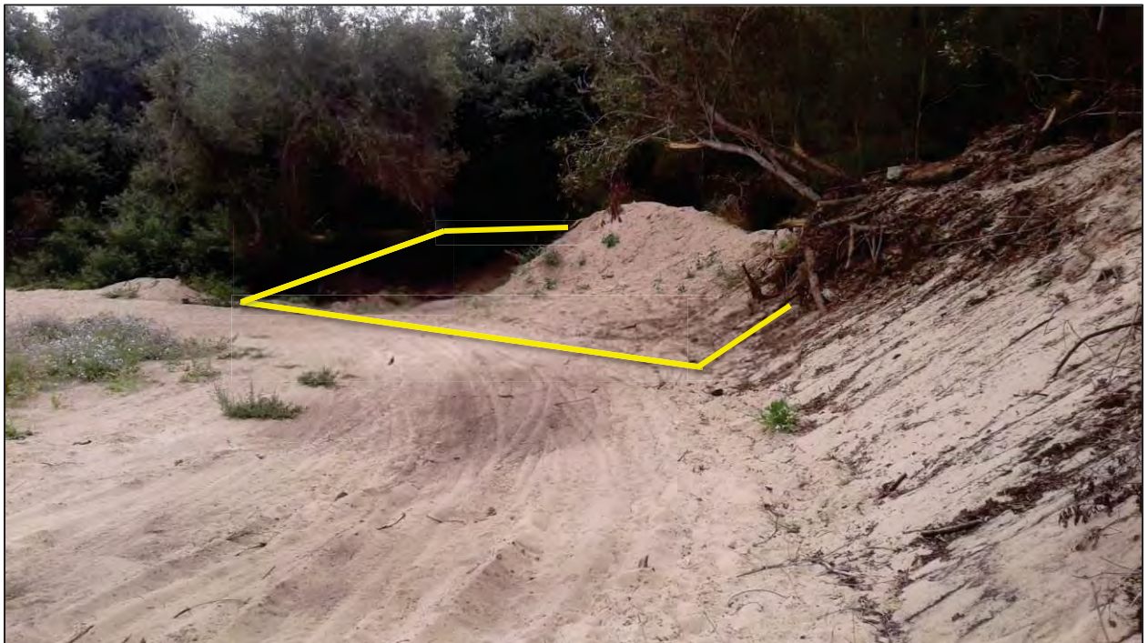
Photo 2. View of the sand that was excavated from the slope shown in Photo 1 and the area within the unnamed tributary to Arroyo Grande Creek proposed for restoration (i.e., native seeding and planting and straw wattles).
