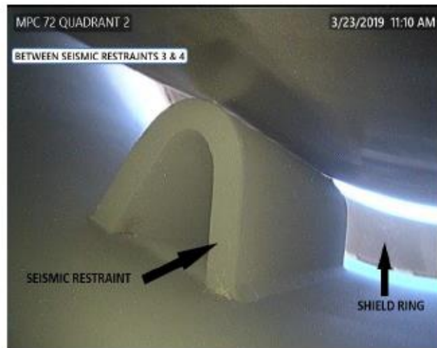
Figure 1. Robotic system photo taken from below the seismic restraint, looking up.
