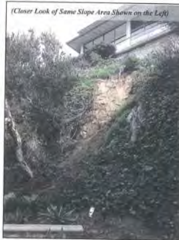
(Slope Conditions below Units 76 to 83; Source : ViaGeos 2017)
