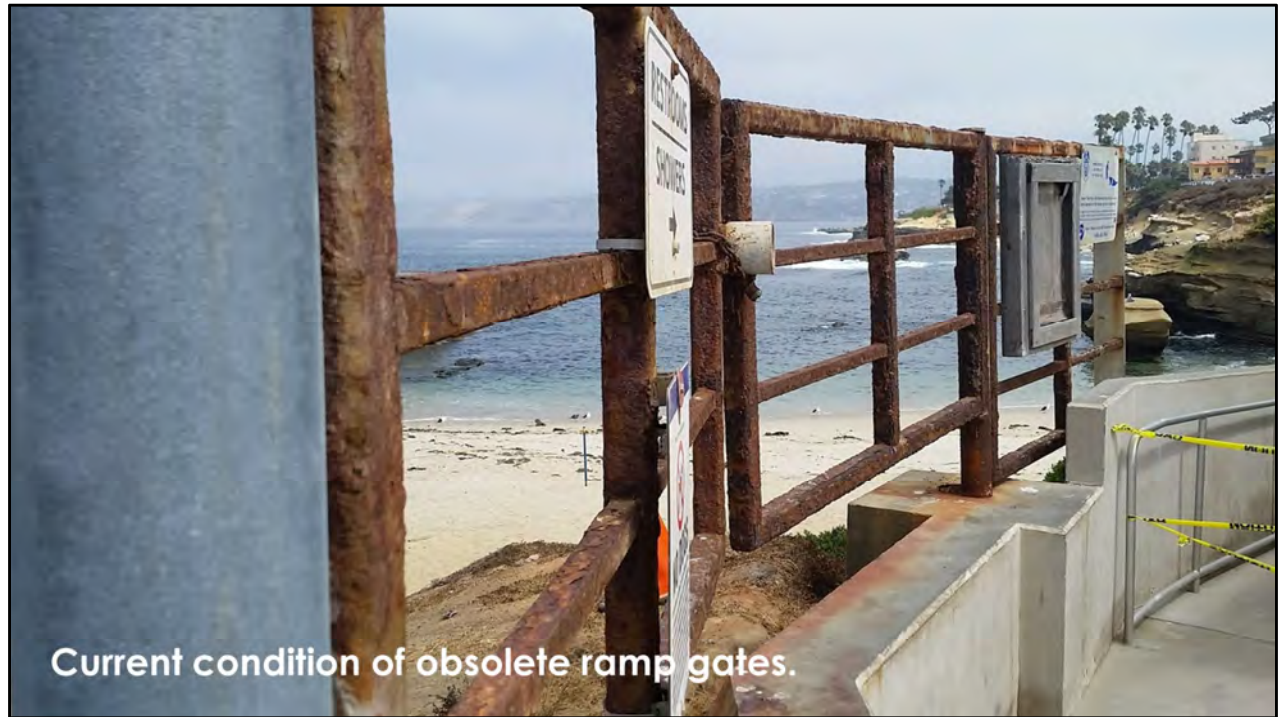
Current condition of obsolete ramp gates. Falling down and dangerous.
