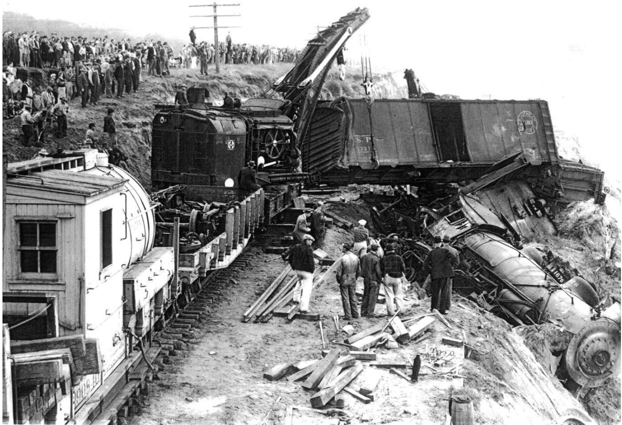
December 31, 1940 bluff collapse and train derailment
