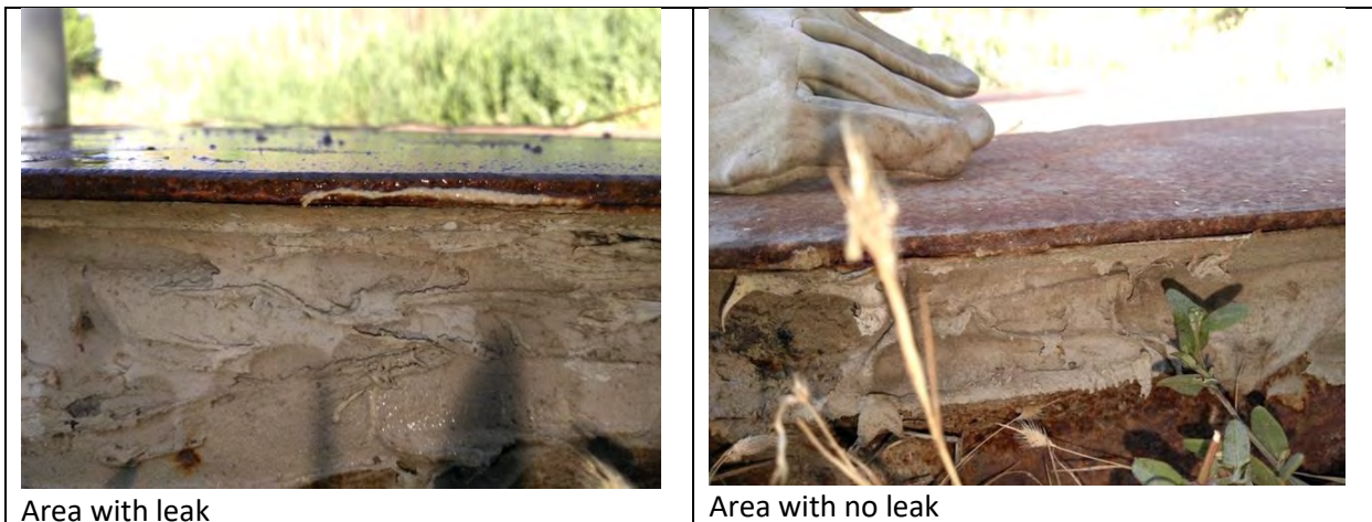
Figure 4: Pictures Meant to Show Difficulty in Finding Any Compromise in the Seal
