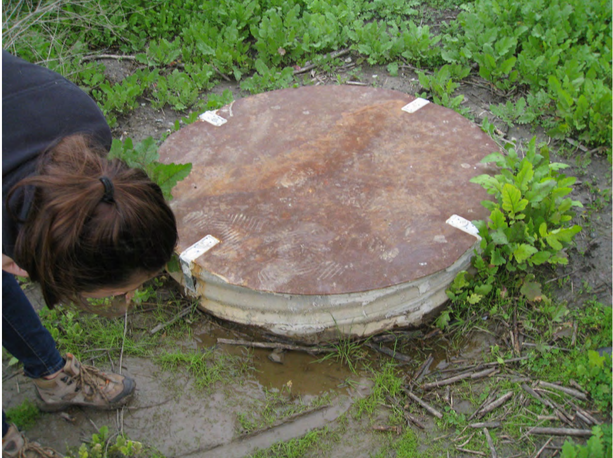
Figure 5. February 1, 2019 photograph of the south drain riser showing small amount of ponded water.
