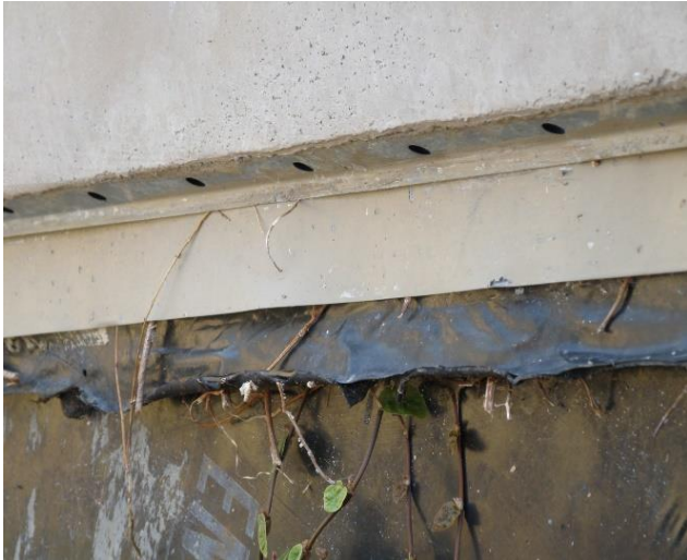
Left: The low-growing groundcover that was planted at the base of the house adjacent to the weep screeds caught on fire. Right: Weep screeds and the frame were repaired and the affected side of the house restuccoed.
