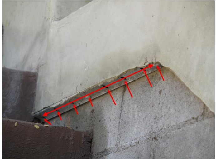
Left: A fire-safe designed home with stuccoed decks and weep screeds protected along concrete steps and concrete exterior flooring (red arrows).
