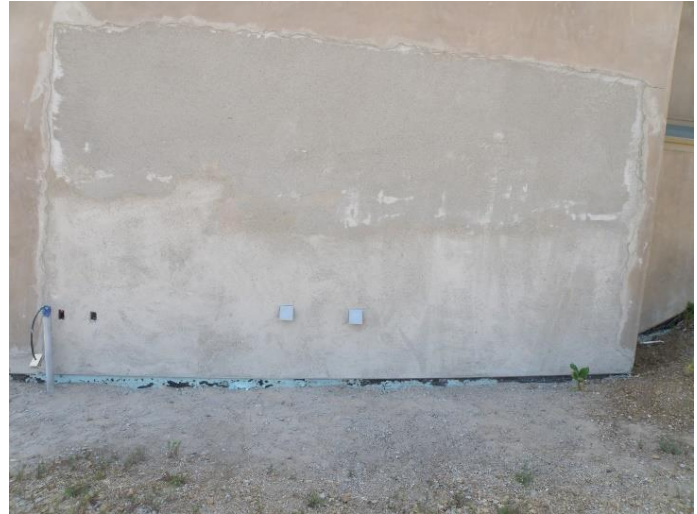
Left: The low-growing groundcover that was planted at the base of the house adjacent to the weep screeds caught on fire. Right: Weep screeds and the frame were repaired and the affected side of the house restuccoed.
