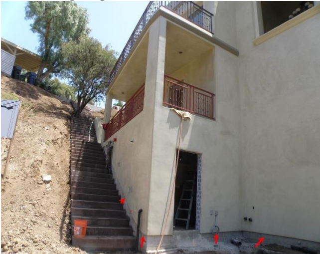
Left: A fire-safe designed home with stuccoed decks and weep screeds protected along concrete steps and concrete exterior flooring (red arrows).
