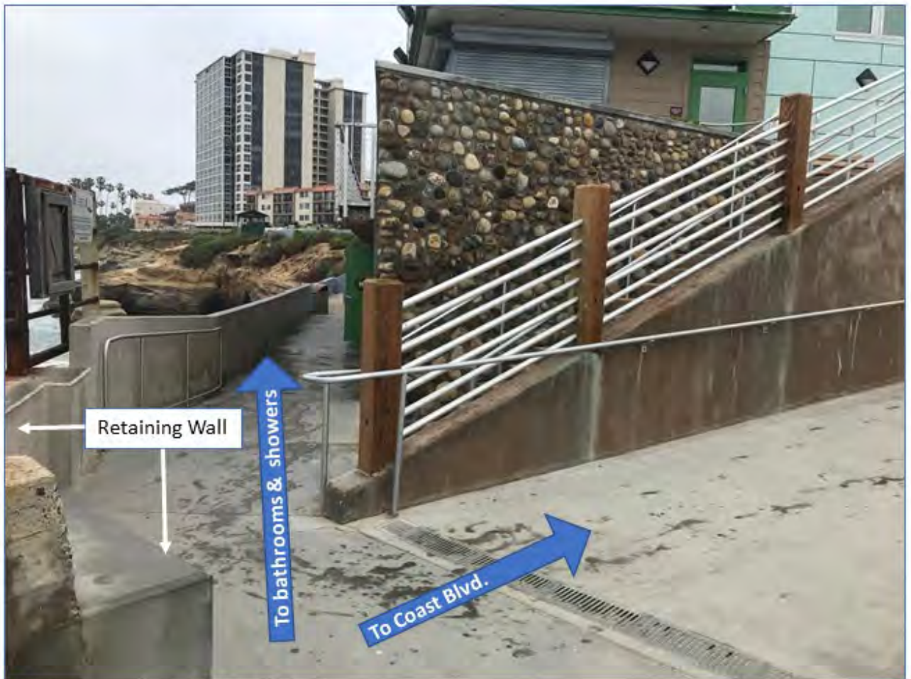
ADA ramp and retaining wall, looking east.
