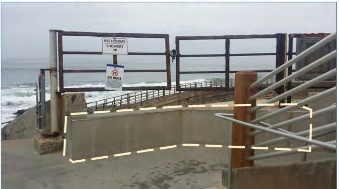
Gate with retaining wall constructed underneath (outlined), looking north.
