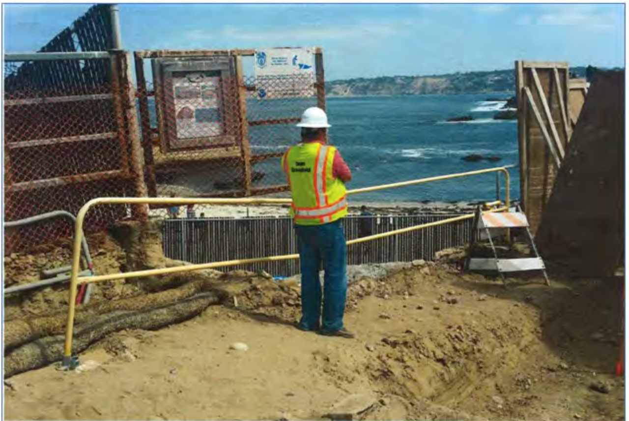
Gate during construction of the lifeguard station, looking north.
