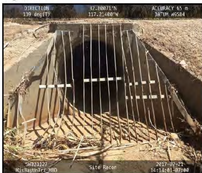
4. Mission Bay Drive 1: Recently maintained culvert inlet at downstream end of segment.
