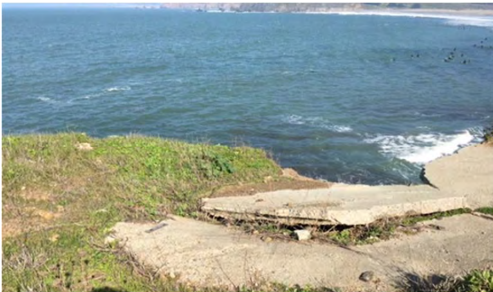
Figure 7: Concrete Slab Falling into Ocean 20 feet from Proposed Development (bluff view)
