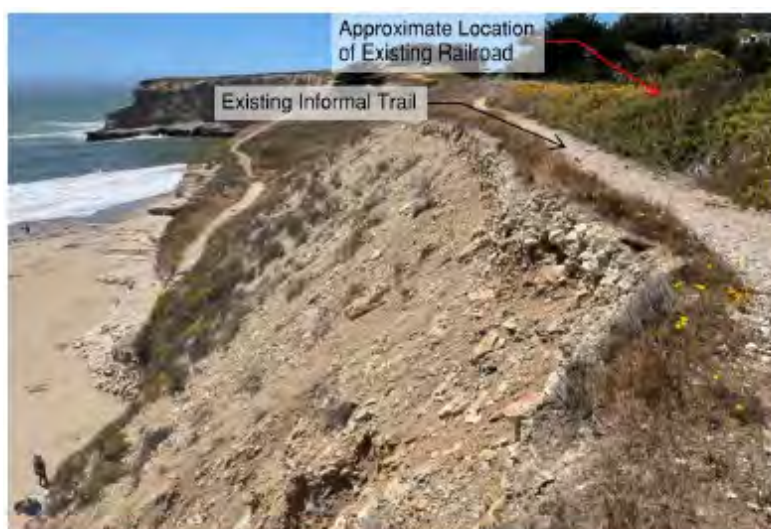
Figure 1: Informal trail and eroding slope. Photo: FHWA.
