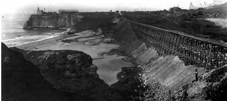
Figure 3: The historic rail trestle and fill at Davenport Beach. Photo: FHWA CD.
