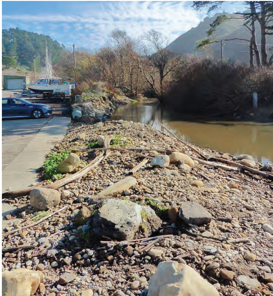
Photo 1: Project area, looking east. Note rocky cobble nature of imported fill to protect parking lot. The sea wall will be constructed along the edge of the existing parking lot. Photo taken January 22, 2020.
