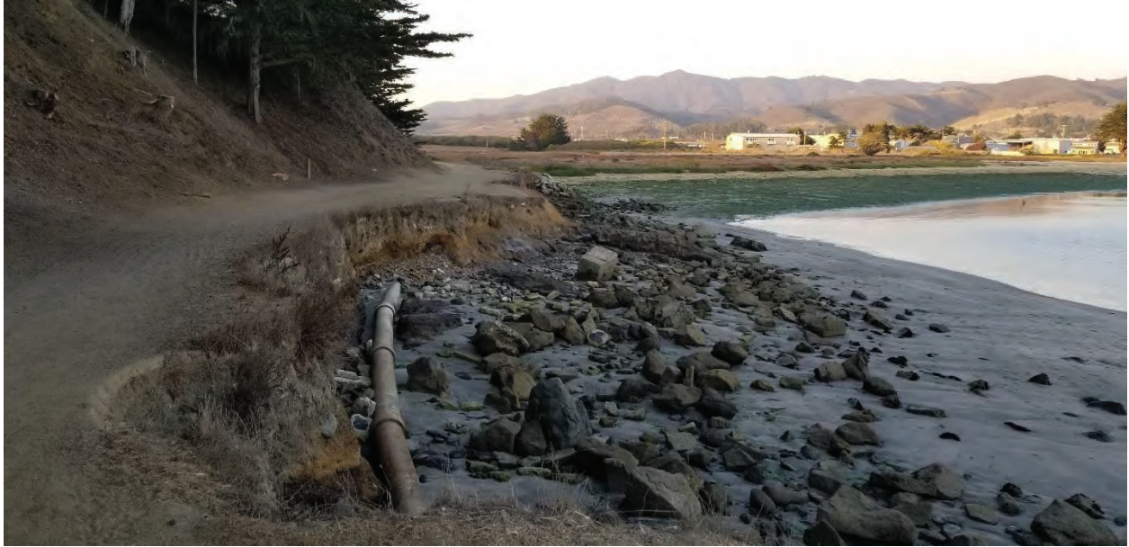
Figure 7. Abandoned asbestos pipe to be encased in cement and sand slurry mix.
