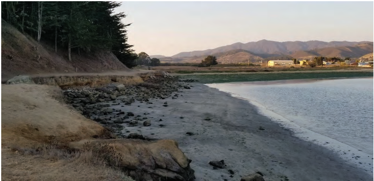
Figure 2. View of undercut trail and rock debris heading north to West Trail parking lot.
