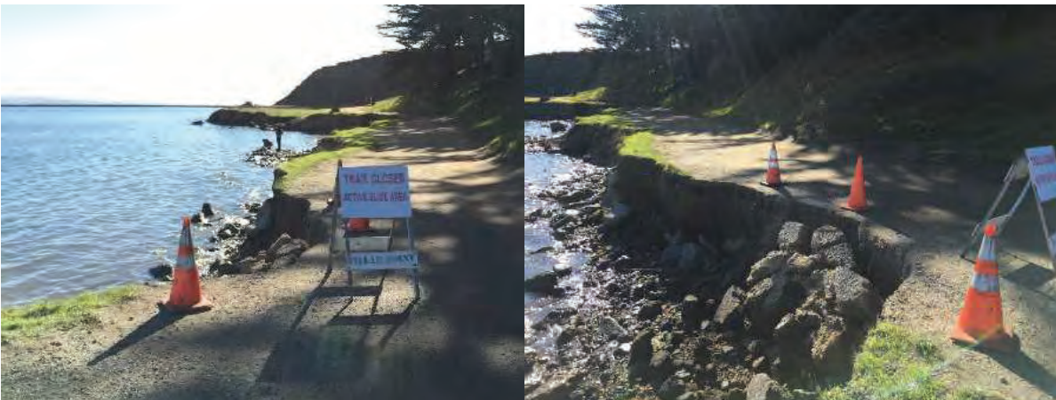
Figure 8. Photos of erosion and trail closures at the West Trail following storms in early December 2019.
