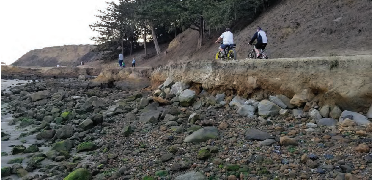
Figure 5. Rock debris next to eroded West Trail being used by pedestrians and cyclists.
