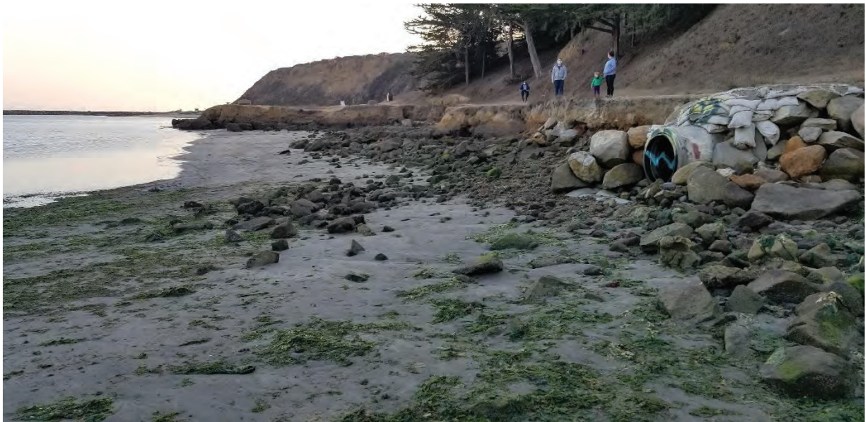
Figure 6. Existing stormwater discharge pipe (to the right of center) with sandbag protection emptying into harbor.
