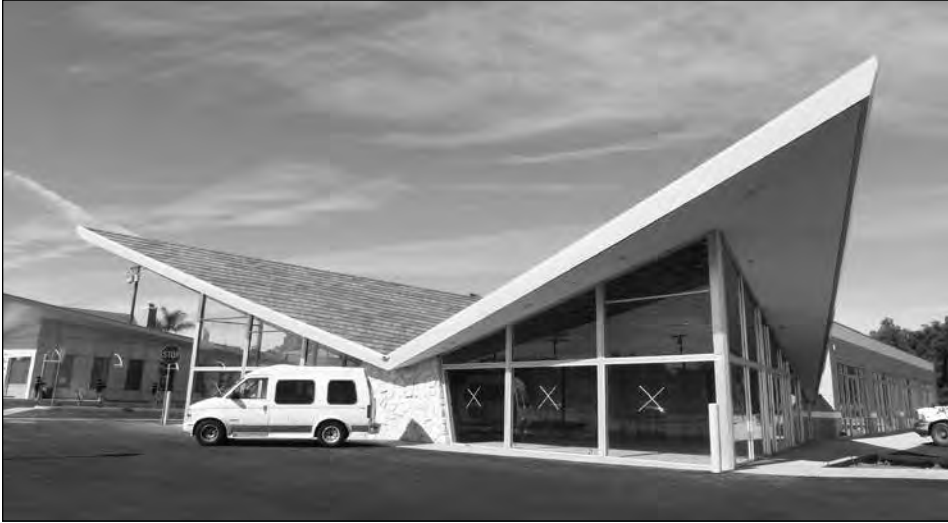
The former Ray Vines Chrysler Agency at the northwest corner of Lakewood Boulevard and Willow Street.
