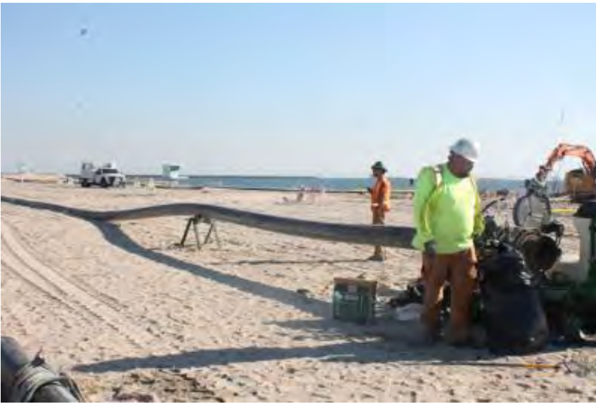
Crews monitor a pump and pipeline last February at the beach near 55th Place. photo by Harry Saltzgaver
