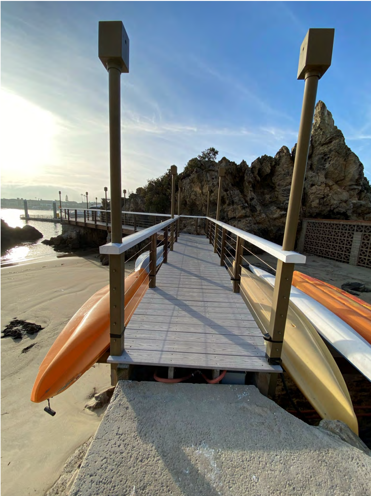
Photo 2: View of Pier from Carnation Cove to Floating Dock
