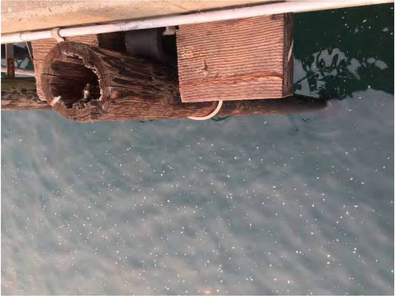
Photograph 4: Another example of a wooden pile that needs replacement on the Arena Cove pier, with aquatic habitat below.
